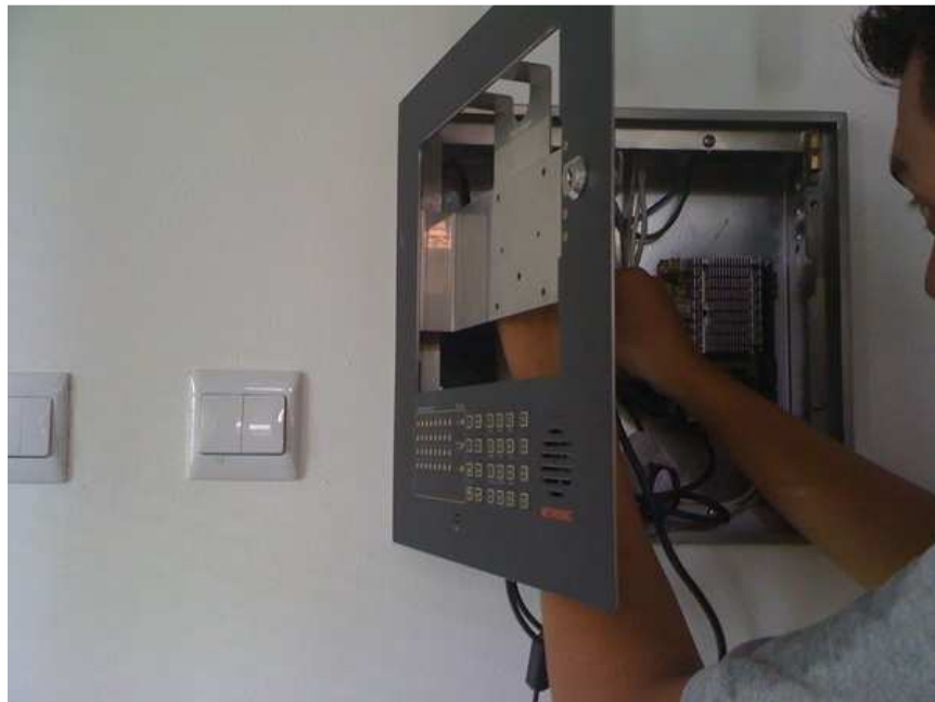
Image 10: Troubleshooting touch panel display for smart home system
